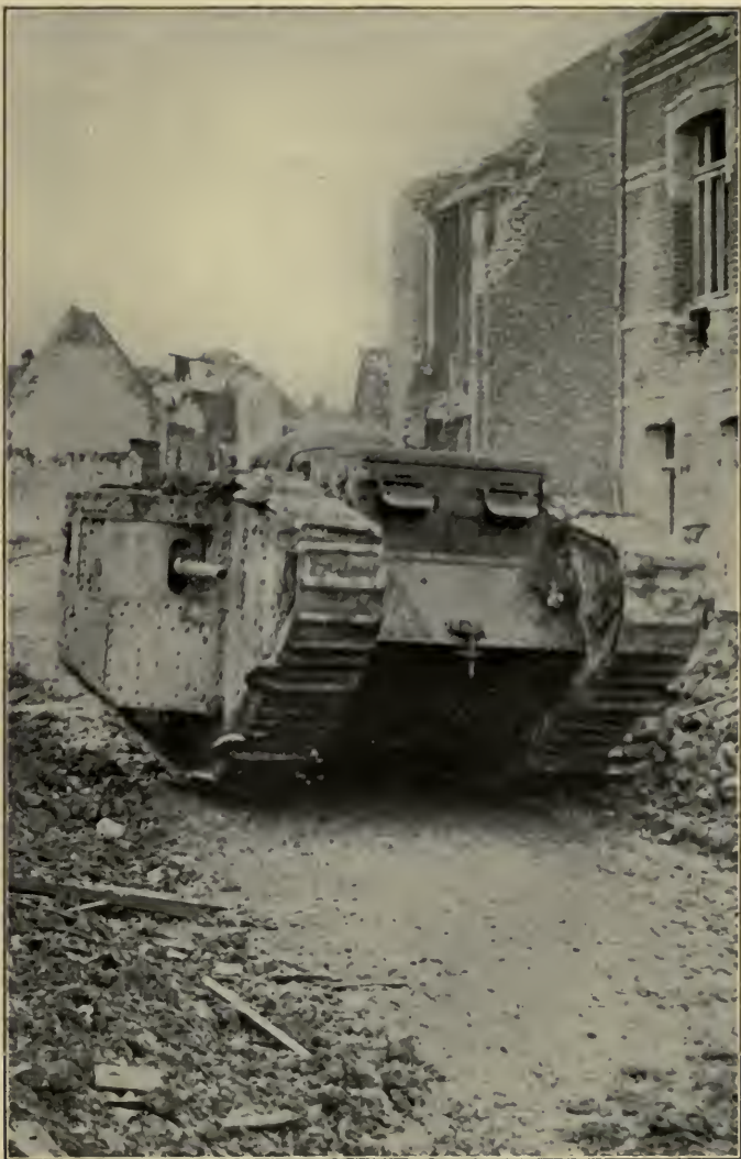
A TANK MOVING TO THE ATTACK DOWN WHAT WAS ONCE A MAIN STREET
